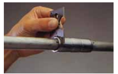
Verify completed joint using same insertion gage.
